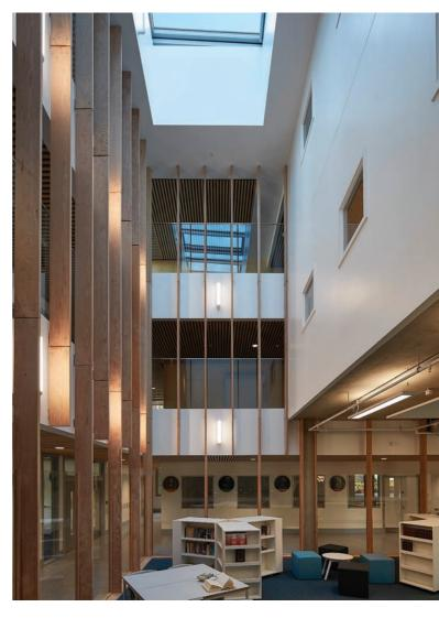
LAMILUX worked with main contractor Willmott Dixon to achieve the required light and solar performance. The triple glazed rooflights were specified with a toughened neutral high performance coated outer pane to provide comfort within the building, whilst achieving impact safety to CWCT TN92 Class 2 U-values and air-tightness values, according to the Passivhaus certificate — verified during the detailed design phase of the project.
